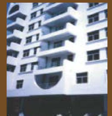
This is a 1994 UNIDO/MRB project. The apartment was the first building in China installed with HDNR bearings designed and fabricated in Malaysia.
