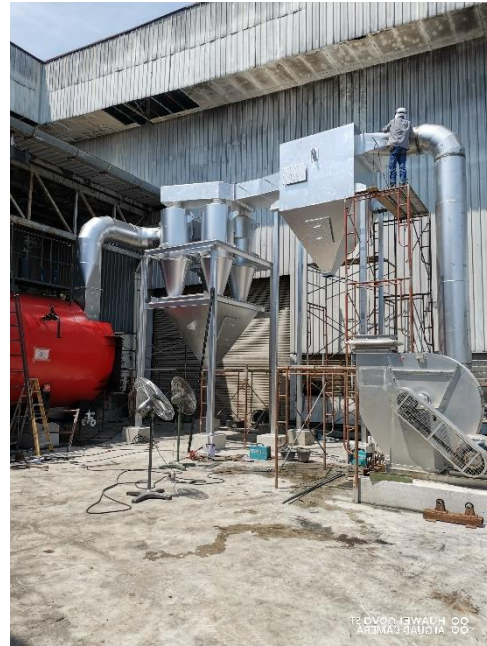
BIOMASS BOILER INSTALLATION
